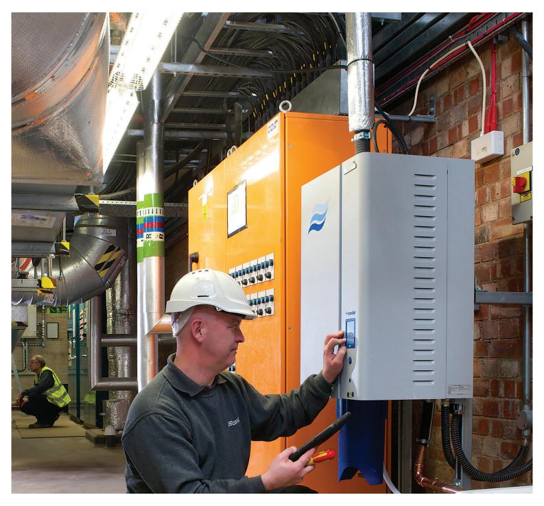
he most common humidifier any HVAC contractor is going to come across is a self-generating, electric steam humidifier. These will typically provide steam to an air handling unit but are also available for direct room humidification with a fan unit. However, for the sake of this guide, I'm going to focus on AHU humidification, as this is the most common.
